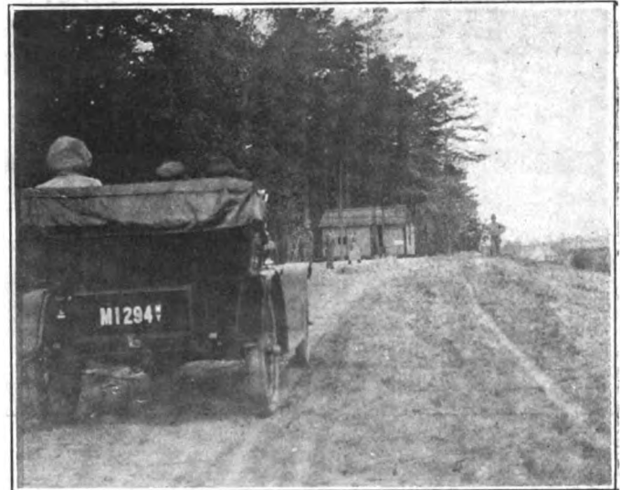
Widening and standardizing the road from Glover to Blacksburg
